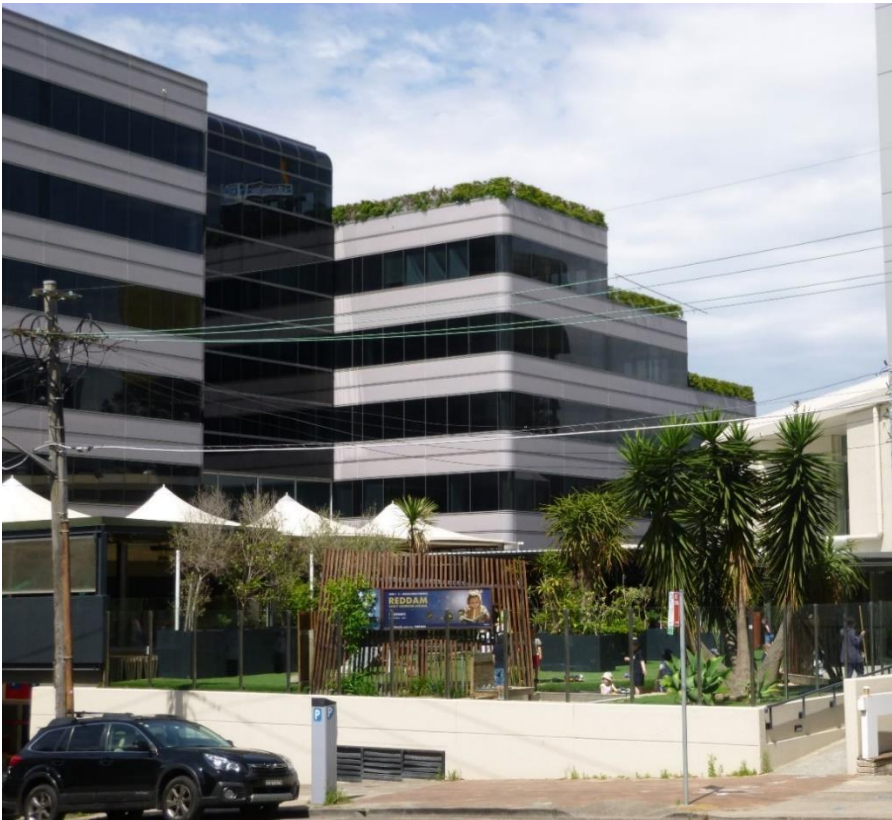
Figure 14. Existing child care centre to the immediate south of the site. The rear portion of the child care centre would be leased by the developer as a site office during construction.
