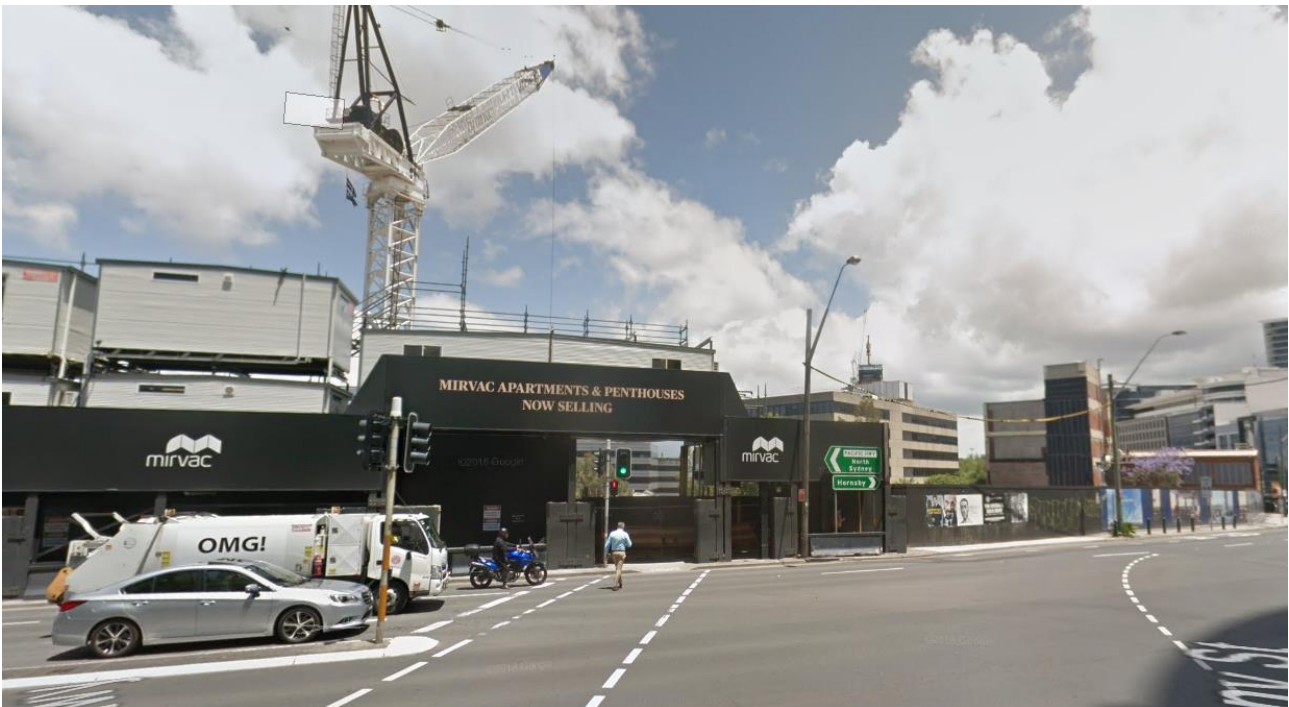
Figure 13. Mirvac and Newhope sites under construction to the east of the site with frontage to Pacific Highway.
