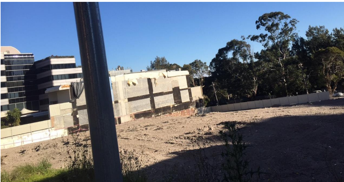
Figure 7. Demolition of the existing buildings (foreground) on 'Site A' and 'Site C' fronting Christie Street and Lithgow Street.
