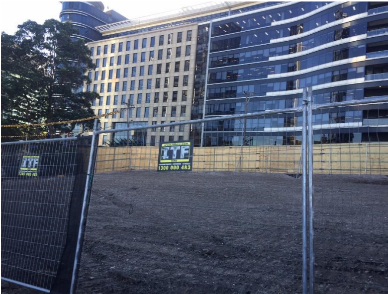
Figure 6. Demolition of existing buildings (foreground) at 564, 562, 560, 558 and 554 Pacific Highway closest to Lithgow Street on 'Site B'.
