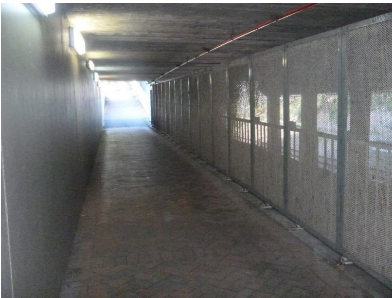
Figure 18. Underground connection at its southern end (Lithgow Street). Lift and stair access are provided at the connections northern end.
