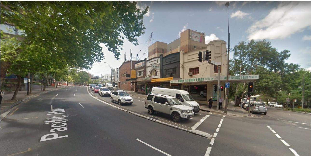
Figure 12. Existing 2-storey commercial development to the east of the site fronting the Pacific Highway.
