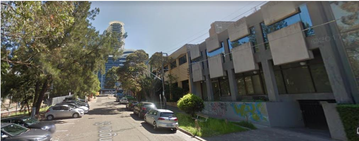
Figure 8. Previous buildings fronting Lithgow Street, now demolished under DA 149/2017.
