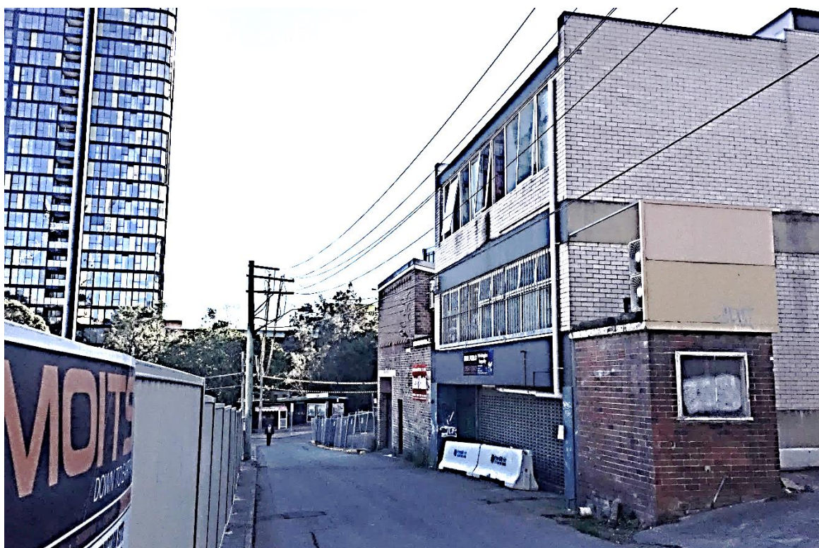
Figure 5. Existing Christie Lane as viewed from Christie Street, and rear of No 546, 548-550 and 552 Pacific Highway. Christie Lane is used by pedestrians to access the Lithgow Street connection to St Leonards train station. This is proposed to be closed during construction. Christie Lane is proposed to be embellished under the VPA providing a through-site link.
